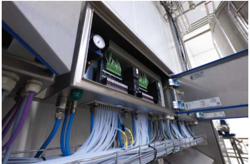
Figure 4: Electrical cabinets are designed to enclose and protect industrial controls for a variety of environmental challenges including dust and water. (Source: Rittal)
